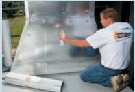
All surfaces should be clean, dry and warm. Use MFM Spray Adhesive™ to improve adhesion in shaded/shadowed areas, on the bottoms of ducts, and in cool temperatures.
