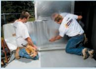
After measuring and cutting the section to the proper size, align and gently press FlexClad into place; reposition if necessary.
