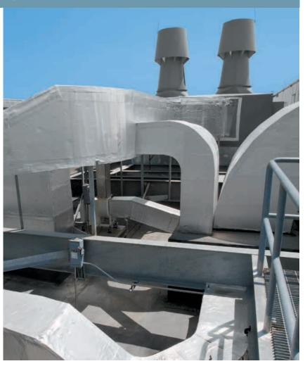
FlexClad can be applied to virtually any shape or configuration. It completely protects the ductwork from infiltration of outside moisture and harmful sunlight, and is warranted by MFM for 10 years.
