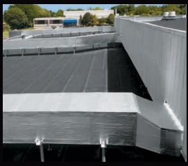
For straight, long length duct systems, FlexClad makes for a clean, uncluttered appearance. Quickly and easily installed, it replaces expensive and cumbersome metal jacketing commonly used to protect insulated ductwork.
