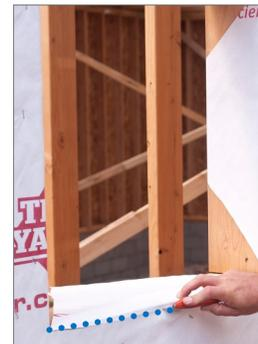
Cut the sill section flush with the bottom of the rough opening and discard.
