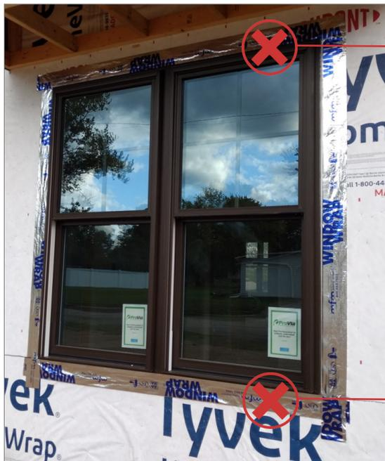
**House wrap was wrapped inside the structure. If water penetrates behind the house wrap, it can funnel right into the structure.**
