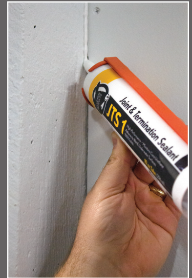
Sealing a joint with white JTS 1 joint and termination sealer.
