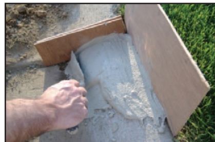
APPLY SPEED MIX TO SUBSTRATE TO BE REPAIRED.
