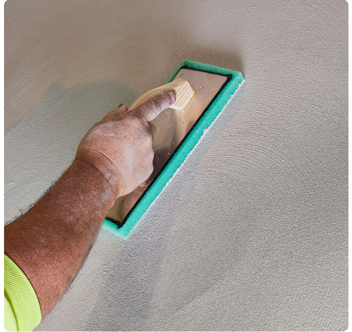
Finish (second) coat (Smooth or Texture Finish)
