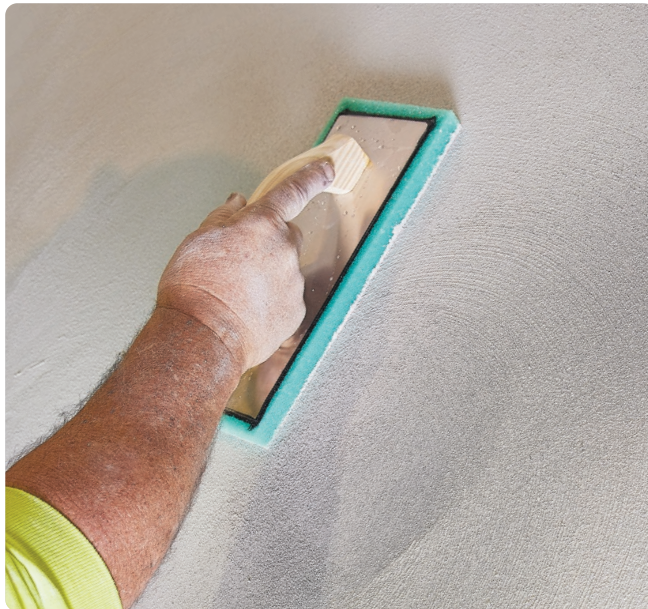
Finish (second) coat (Smooth or Texture Finish)
