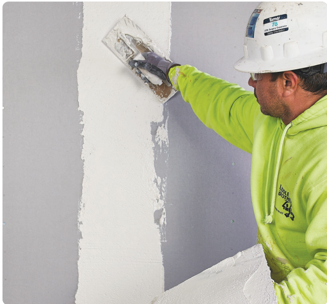
Base (first) coat on Kal-Kore Plaster Base
