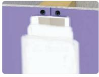
Additional coating of compound over joints and interior angles. Smooth and free of tool marks and ridges.
