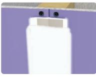
Thin coating of compound over all joints and interior angles.
