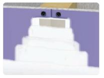
Skim coat applied over entire surface. Surface smooth and free of tool marks or ridges.
