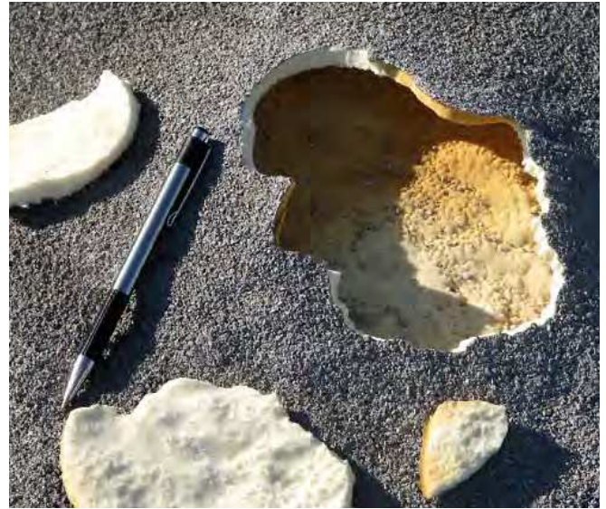
Foam blister that has been cut open
