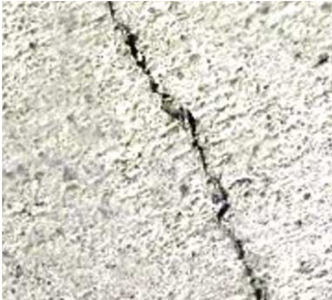
Crack before coating
