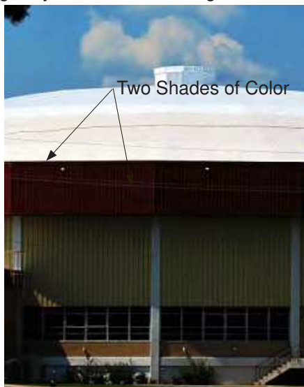
Roof with moisture contamination
