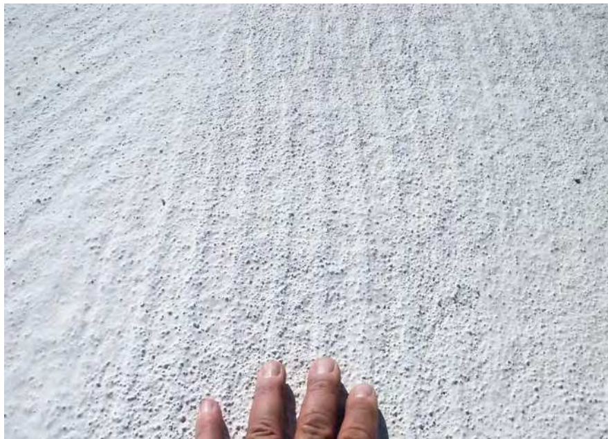
Coverage rates and aggregate distribution is inconsistent
