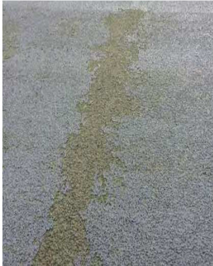
Delamination due to incompatible materials
