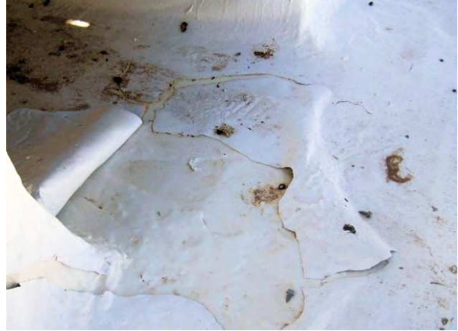
Delamination due to improper cleaning
