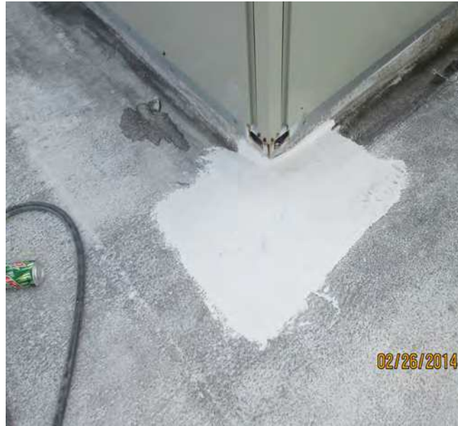
Area was not cleaned prior to repair.
