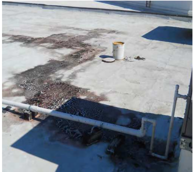
Poorly maintained condensate drain lines results in contaminated coating.
