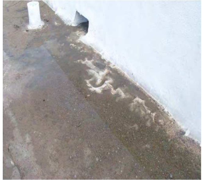
Topcoat delaminating from ponding due to clogged roof drain.
