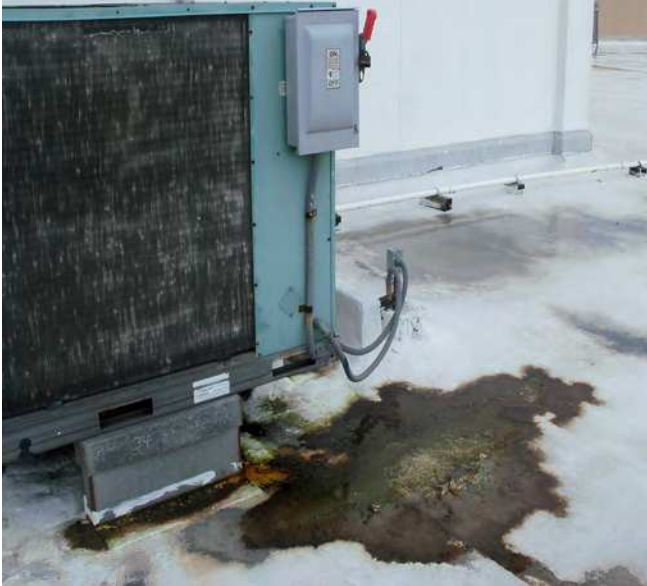
Disconnected condensate drain lines contaminated coating.
