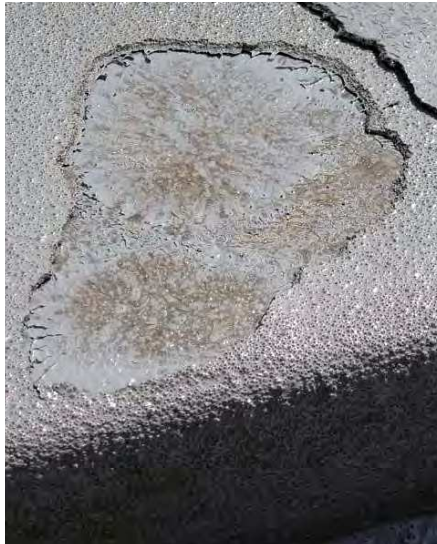
Area underneath removed blister
