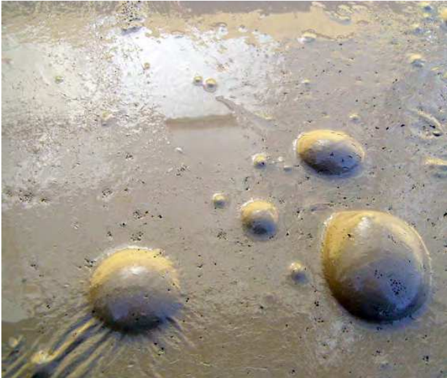
Blisters from rain/sprinkler system
