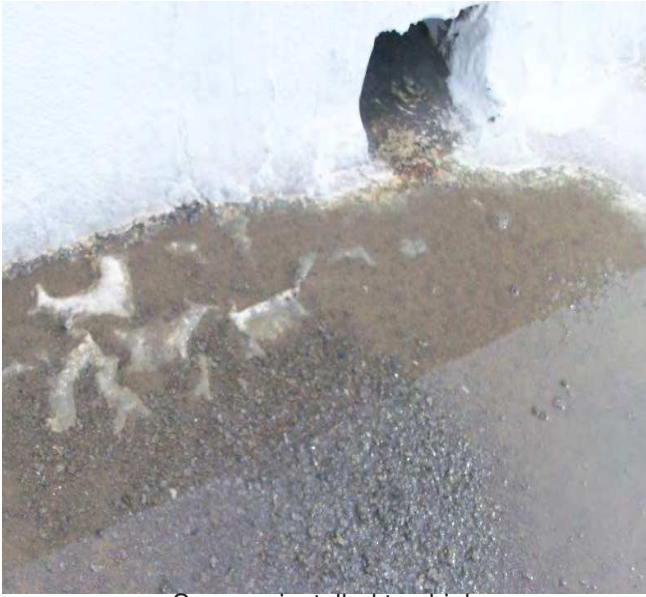
Scupper installed too high
