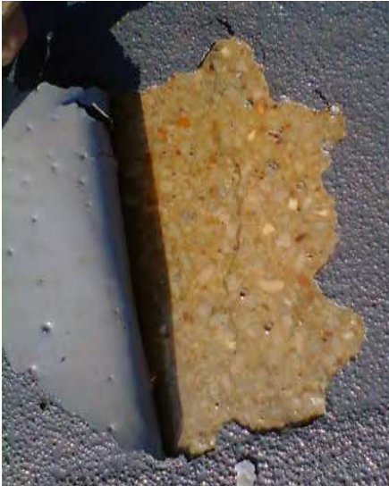
Delamination due to moisture
