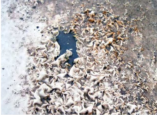
Delamination due to thin topcoat and ponding
