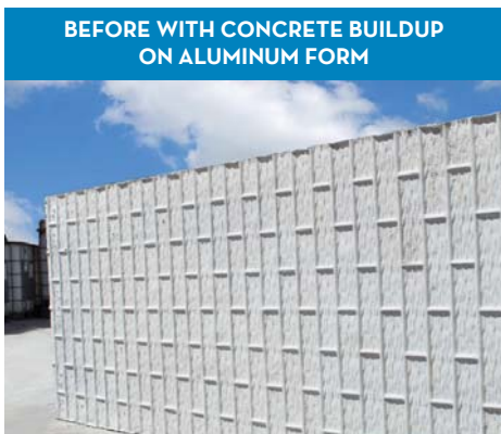
BLAST-OFF ON ALUMINUM FORMS
