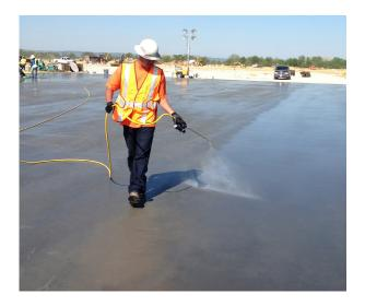
Silcoseal Select, Silcoseal 2000F, and Silcoseal Classic all met the ASTM C309 72-hour moisture loss benchmark of 0.55 kg/sm when applied to a concrete surface finished with a steel trowel under the guidelines set forth in CEN/TS 14754.
