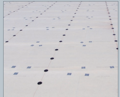
2. Secure a cover board* to the purlins with RetroDriller fasteners and round RhinoBond Plates for membrane attachment. *Additional non-RhinoBond insulation fasteners may be required per FM guidelines, as illustrated by the square plates shown above. Spacing is always specified by the roof system manufacturer.
