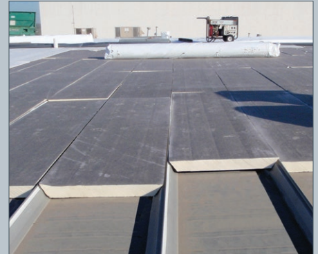
1. Fill the flutes with tapered insulation.
