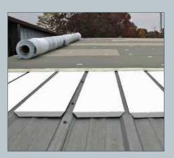
RhinoBond is also an ideal option for metal roof retrofit applications. Because the system does not require in-seam fastening, and the membrane seams do not have to be positioned over the purlins. This eliminates the need for specialty purlin-width sheets, simplifies the installation, reduces waste, and can improve productivity.
