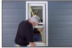
**Apply OSI® QUAD® foam** into the gap between the pocket window and the framing at the head and side jambs. Do not apply foam between the pocket window sill and the window sill.
