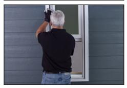
Apply flashing tape to the window sill, butting it up to the interior stop. Flashing tape should measure the same width of the window frame and the depth of the replacement window frame. Use the J-roller to remove any air pockets.
