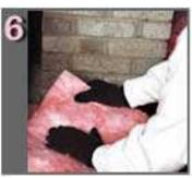
Around masonry chimneys or other areas that have small openings, stuff these spaces with small pieces of unfaced insulation, which will not burn.
