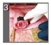
If the joist cavities are completely filled, lay the new insulation in long runs perpendicular to the direction of the joists, and use leftover pieces for small spaces. If the cavity is not completely filled, use the appropriate thickness of insulation to fill it to the top, then add an additional layer of insulation in the perpendicular direction.
