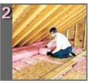
Lay the insulation blanket at the outer edge of the attic space and work toward the center. This allows for more headroom in the center of the space, where cutting and fitting can be done. It's also a good idea not to get "insulated into a corner" where it will be hard to get back to the attic entry way.
