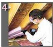
The insulation should extend far enough to cover the tops of the exterior walls, but should not block the flow of air from the eave vents. To make sure the eave vents aren't blocked, Owens Corning Raft-R-Mate® attic vents or baffles should be installed to provide unrestricted air flow from the soffit to the attic.
