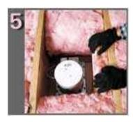
Insulation should be kept three inches away from recessed lighting fixtures unless the fixture is marked "I.C." (Insulated Ceiling), which is designed for direct contact with the insulation. If insulation is placed over an unrated fixture, it may cause the fixture to overheat and perhaps start a fire. Also, the insulation should always be installed at least three inches away from any metal chimneys, gas water heater flues or other heat-producing devices.
