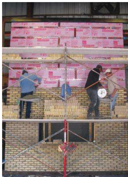
NFPA 285 test wall under construction.
