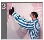
With either faced or unfaced insulation with a separate polyethylene vapor retarder, an interior finish material, such as drywall, should be installed as soon as the insulation is in place.
