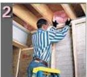
For the band joist, use unfaced cut-to-fit pieces of insulation and place them snugly into the space. If a vapor retarder is needed, cut poly to fit over insulation.
