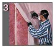
If unfaced insulation is used for basement walls, a 4- to 6- mil poly vapor retarder will need to be installed.
