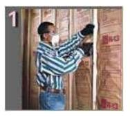
Either faced or unfaced exterior wall insulation can be used on basement walls, with R-values ranging from 11 to 21. Faced insulation should be placed between the studs with the vapor retarder facing the interior of the room in heating climates. The flange on the facing can be stapled to the inside or face of the stud.
