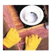
3. Insulation should be kept three inches away from recessed lighting fixtures unless the fixture is marked "I.C." (Insulated Ceiling), which is designed for direct contact with the insulation. If insulation is placed over an unrated fixture, it may cause the fixture to overheat and perhaps start a fire. Also, the insulation should always be installed at least three inches away from any metal chimneys, gas water heater flues or other heat-producing devices.
