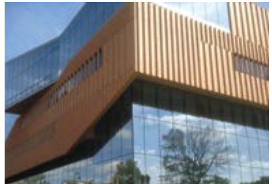
Solutions | Improve Acoustics, LEED® Platinum Certification
