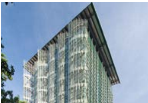
Solutions | Fire Safety, LEED® Platinum Certification
