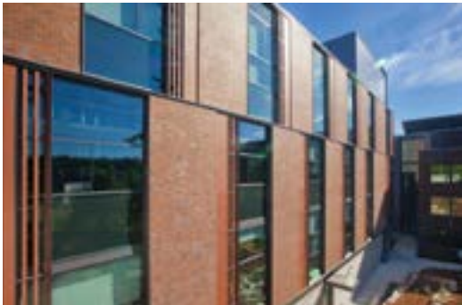
Solutions | Maritime Climate, LEED® Gold Certification
