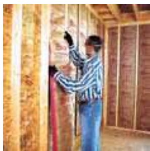
1. For standard wall heights, use pre-cut batts rather than continuous rolls. Each piece of insulation is manufactured to the size of the most typical framing, which usually is built either 16 or 24 inches on center and about 92 inches high. These cut-to-size batts will make the job go faster and easier. *MIRAFLEX®* R-13 insulation comes with a poly facing and is ideal for exterior walls. It features a poly wrap over the *MIRAFLEX* fiber batt on three sides so it's easy to handle and install.
