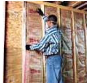
Note: Never leave faced insulation exposed. The facings on Kraft-and-foil-faced insulation will burn and must be installed in substantial contact with an approved ceiling, wall or construction material to help prevent the spread of fire in the wall, ceiling or floor cavities. Unfaced fiber glass is non-combustible.
