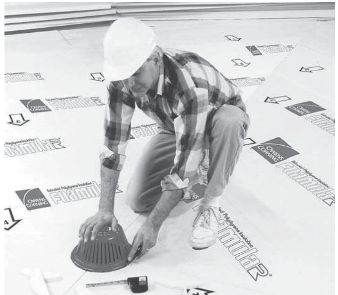
Typical Tapered Roofing Section, 1/8" per foot slope
