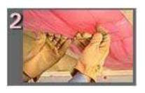
Insulation will stay in place temporarily if you are using R-19. R-25 insulation needs to be supported as you go. Use metal insulation supports (16" or 24" wire rods or crisscrossed wire) to hold insulation in place. Be careful not to compress insulation too much with supports. Insulation should fit snugly against band joist and overlap bottom plate.
