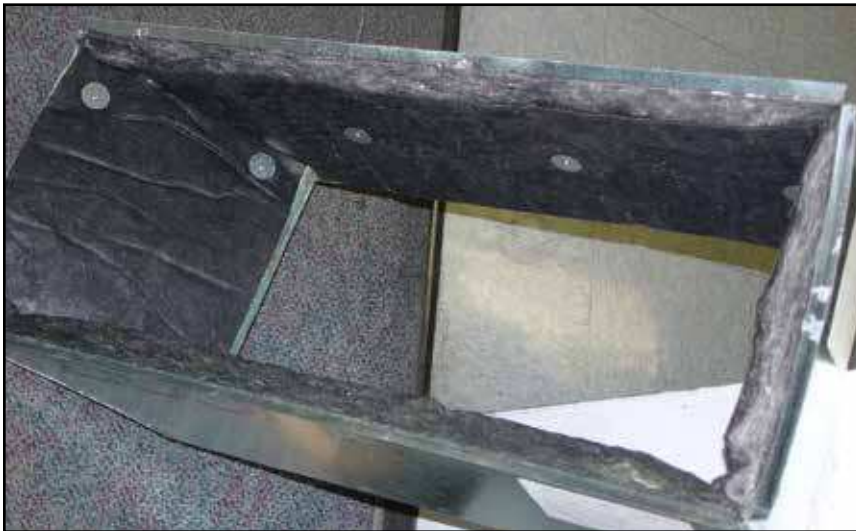
Figure 32 - Insulated diffuser box
