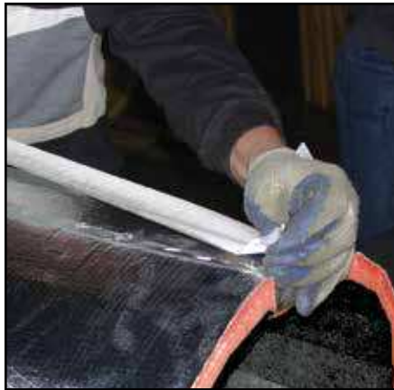
Figure 5 - Stapling and taping
