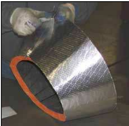
Figure 28 - Assembling reducer
