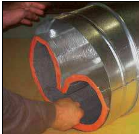
Figure 16 - Inserting gore into elbows
