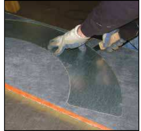
Figure 24 - Cutting sides at an angle
