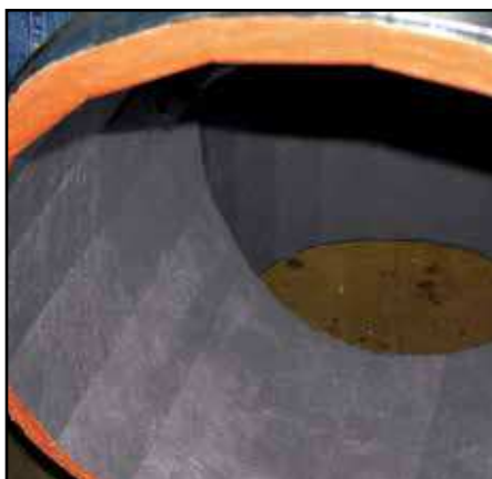
Figure 21 - Finished edge of Tee
