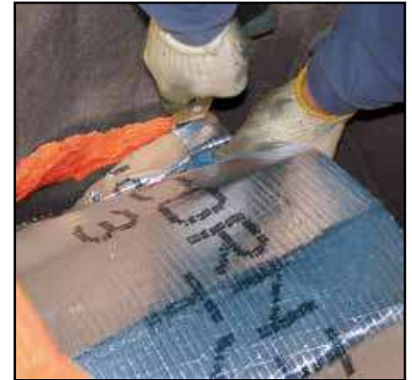
Figure 20 - Trimming straight leg of Tee
