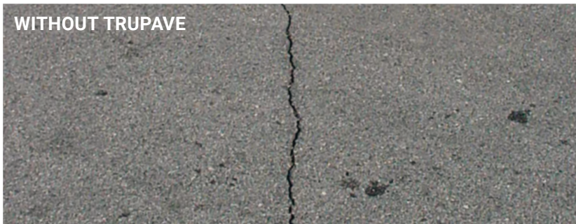
Lakeland, FL: Installed February 2001 Soil Cement Base | Overlay over HMA | Cracking stops at TruPave
