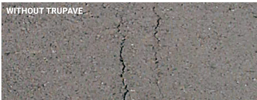
Texarkana, AR: Installed December 2001 Unknown Base | Overlay over PCC | Cracking stops at TruPave
