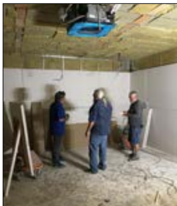
Full Exposure: QuietRock 545 installation over steel framing
