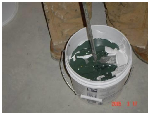
Photo #15 – Sealant Mixing in Process
