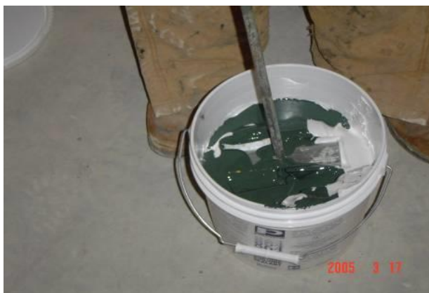
Picture #15: Sealant Mixing in Process
