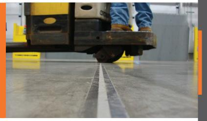
PNA has been helping to reduce floor maintenance costs by eliminating joint spalling for over 20 years with Armor-Edge. It has proved itself an ideal solution for construction joints in speed aisles, door thresholds, high-traffic areas, and freezer (cold storage) facilities.
