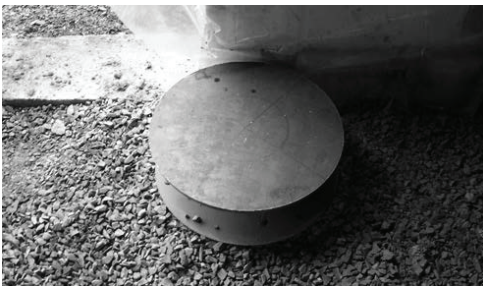
PNA bollard base on level subgrade
