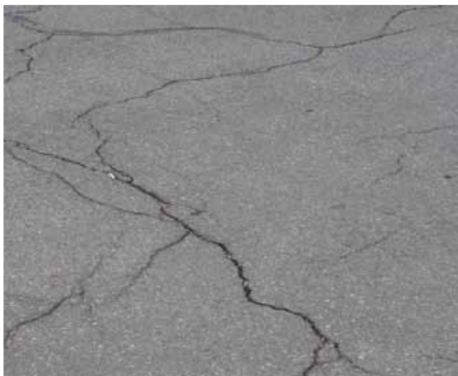
Figure 15b. Low- to medium-severity random cracking
