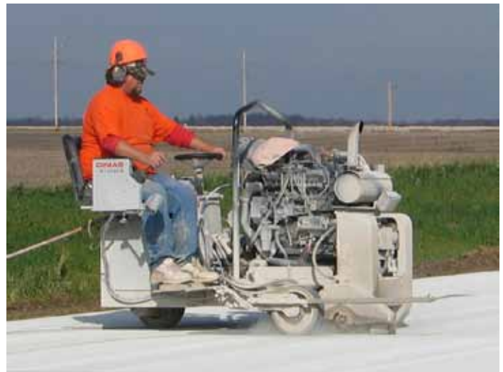
Figure 49. Conventional joint saw
