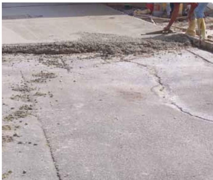
Figure 1. Concrete overlay being constructed over medium-severity block-cracked asphalt parking lot
