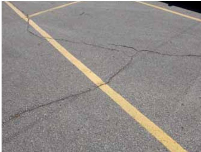
Figure 15a. Low- to medium-severity random cracking
