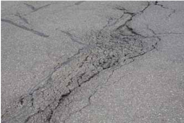
Figure 12a. Low- to medium-severity pothole
