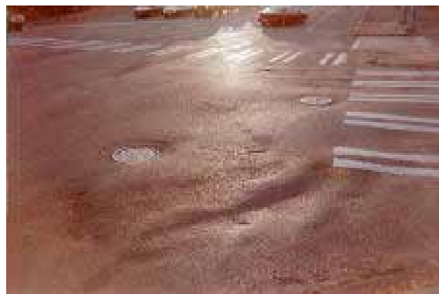
Figure 17b. High-severity shoving
