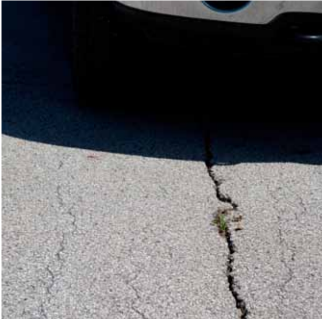
Figure 14a. Low- to medium-severity thermal cracking
