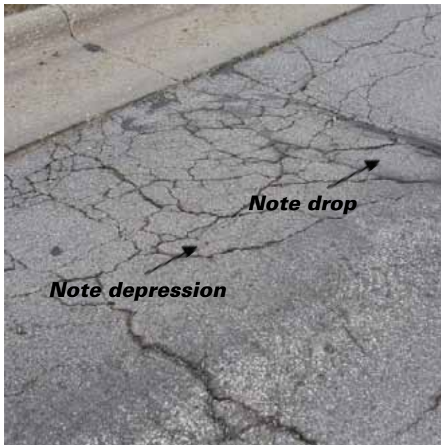
Figure 11b. High-severity block cracking
