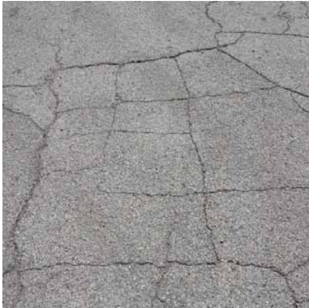
Figure 11a. Low- to medium-severity block cracking
