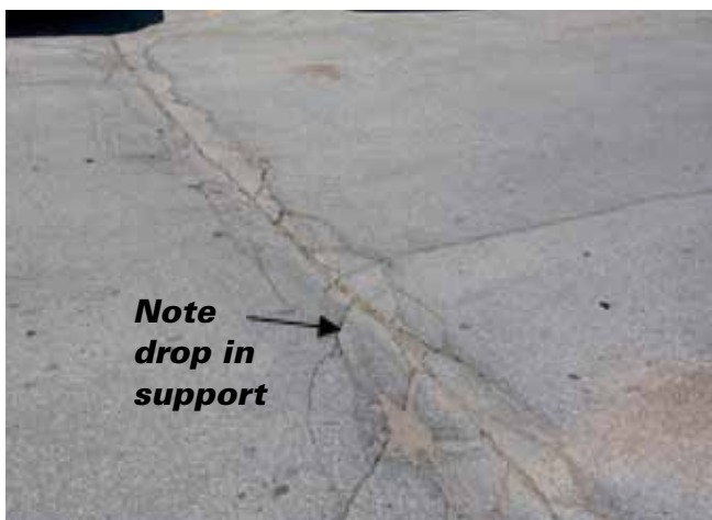
Figure 15c. High-severity random cracking
