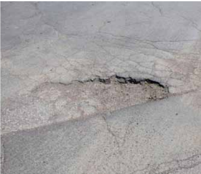
Figure 12b. High-severity pothole
