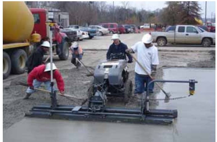
Figure 47. This walk-behind laser-guided screed will pave flat, crowned, or inverted pavements with 3D Profile Package installed; typically used to reach places larger machines cannot
