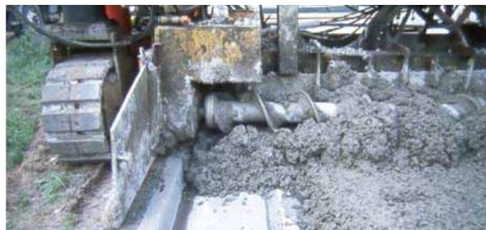
Figure 24. Slipform curb over existing curb
