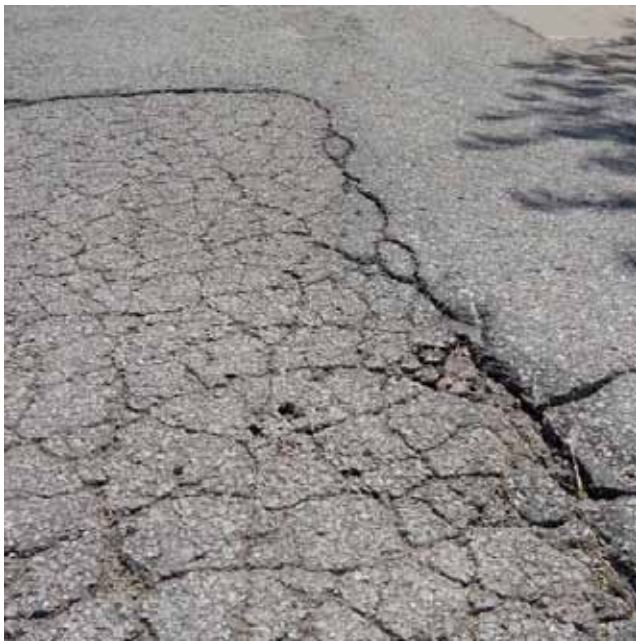
Figure 10b. High-severity alligator cracking
