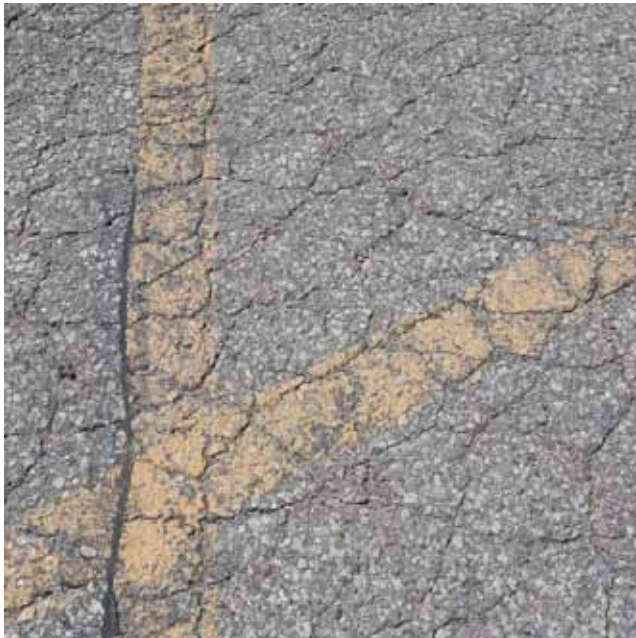
Figure 10a. Low- to medium-severity alligator cracking
