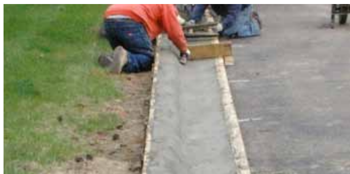
Figure 22. Finishers “capping” existing curb and gutter; the form line is the edge of the asphalt and existing curb, and another form is used at the back of the curb (Photo courtesy of Jim Amundsen, Grace Construction Products)
