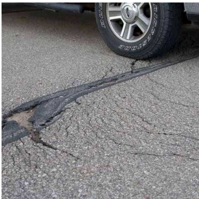
Figure 17a. Low- to medium-severity shoving
