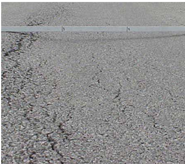
Figure 16a. Low- to medium-severity rutting
