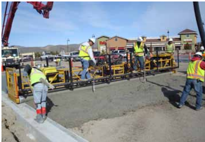
Figure 44. This high production, non-vibrating spinning triple-roller tube paver is used on small, medium, or large projects at paving widths from 10- to 32-ft wide; flat pavements up to 50,000 sq ft/day
