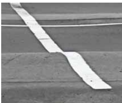
Figure 16b. High-severity rutting
