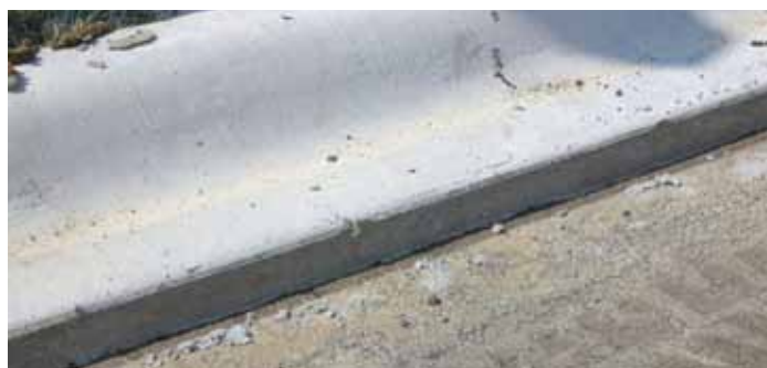
Figure 23. Completed curb section ready for overlay placement
