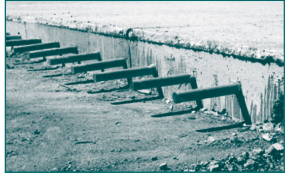
Figure 5. Photo of epoxy-coated dowel bars in full-depth concrete pavement repair (photo credit: www.pavement interactive.org)
