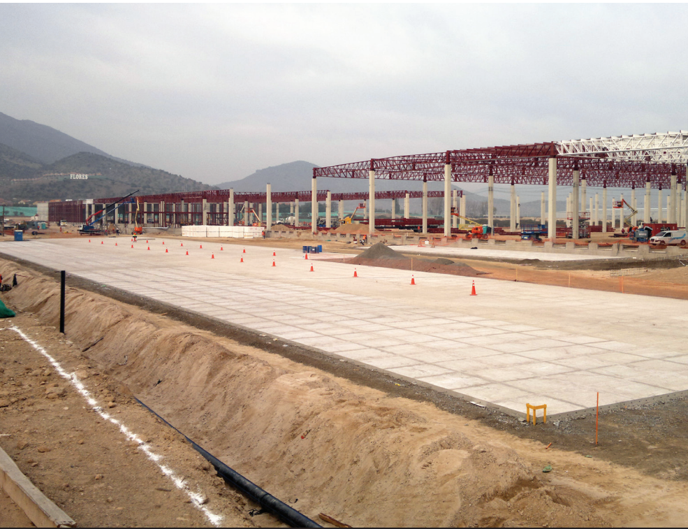
Walmart began using Thin Concrete Pavement (TCP) technology in Chile in 2011.
