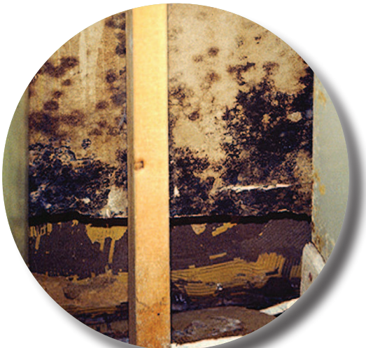
Black mold in wall assembly. Photo courtesy of the American Phytopathological Society
