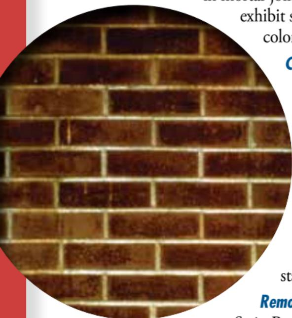
**Cause:** Cleaning with muriatic acid. Acid and impurities in the acid are rapidly absorbed by porous masonry and cannot be thoroughly water-rinsed. As the acid attacks the bricks and mortar, soluble and insoluble salts are mobilized to create unsightly stains.
