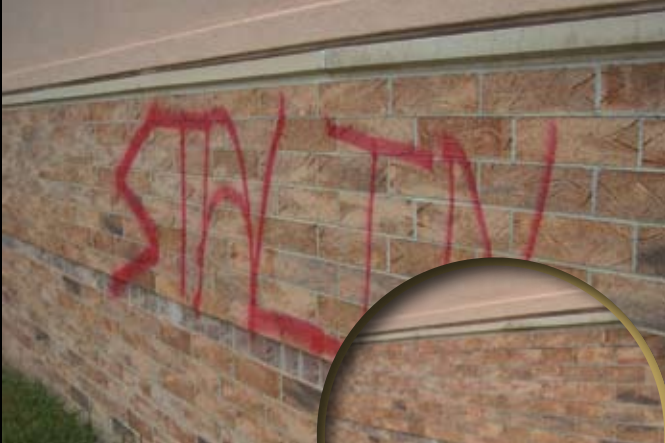
Graffiti removal from brick masonry.
