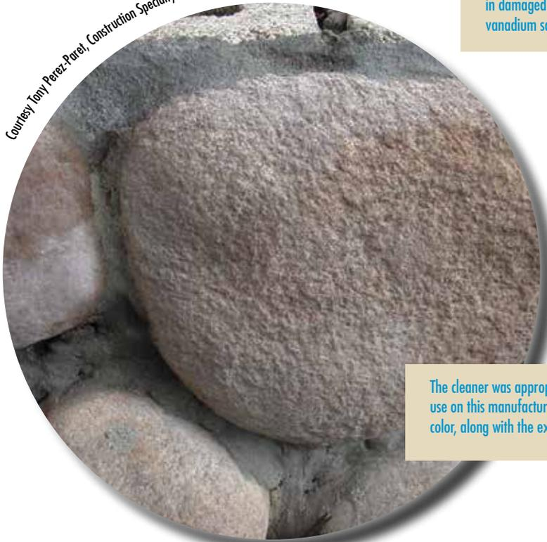
The cleaner was appropriate for clay brick. Unfortunately, the contractor didn't test it before use on this manufactured river stone. The cleaner removed much of the stone's surface-applied color, along with the excess mortar.
