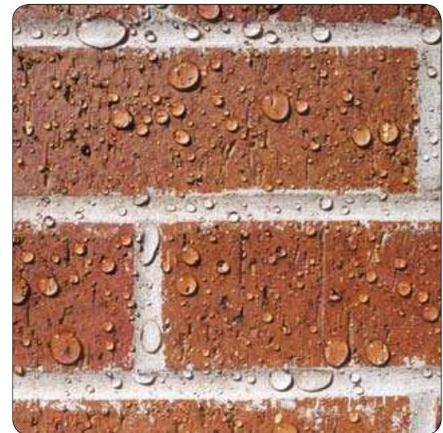
Water beads up and runs off bricks treated with Sure Klean® Weather Seal Siloxane PD.
