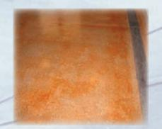
QC CONCRETE DYE penetrates deep into the concrete slab or overlay surface and permeates the pores of the substrate leaving no film or coating to be worn away.
