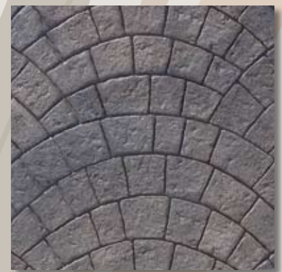
Stone Gray Color Hardener Liquid Release with Blackfoot and Buckwheat Patina Stain
