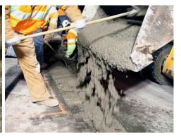
**QUIKRETE® Rapid Road Repair** is a very high strength, rapid hardening material used to make permanent repairs to concrete surfaces. The material is made of specially formulated fast-setting cements and is reinforced with AR glass fibers for improved flexural performance essential for applications of severe vibrations, such as bridge deck repairs.
