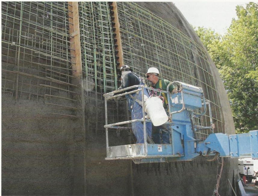
Fig. 2: Wet-mix shotcrete installation at dome structure
