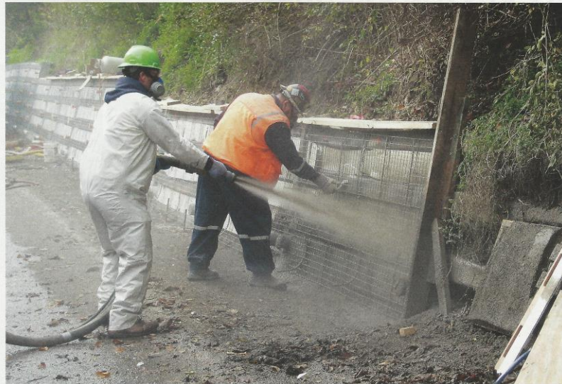
Fig. 1: Dry-mix shotcrete being installed on a retaining wall project
