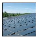
Dura♦Skrim® reinforced sandbags are used to secure large covers and liners to prevent wind damage. Sandbags are produced with strong Dura Skrim® 8 & 12 mil reinforced polyethylene. These 15" wide x 24" long bags are designed to hold 35 lbs. Sandbags are also available in other Raven reinforced materials with minimum order requirements.
