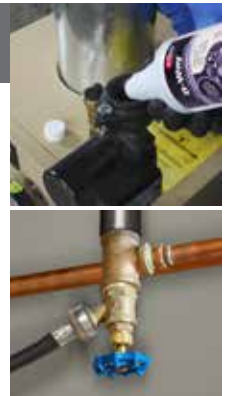
▲ Force pump drain line injection
