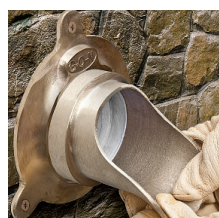
Solvent weld nozzle onto pipe and into escutcheon. Dura G-O-N requires the mounting notch in the escutcheon and the nozzle be aligned for proper contact.
