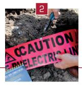
Place one clip on each side of the overlapping sections and crimp each clip securely with pliers.
