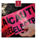
Overlap two ends of detectable tape being spliced by 6-10 inches.
