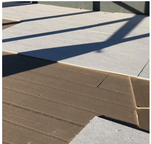
Rmax Ultra-Max® HD is applied above the roof deck and insulation layer to provide a suitable substrate for roofing membranes as well as suitable protection for underlying insulation.
