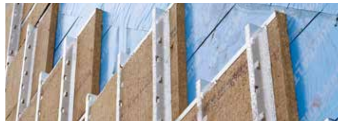
Crossing Z-girt cladding support system with custom punched vertical Z-girt profiles used to retain ROCKWOOL CAVITYROCK® insulation.
