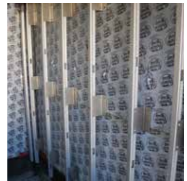
Intermittent stainless steel clips with vertical girts.
