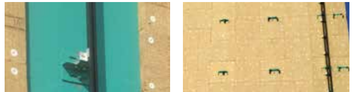
Example of heavy-duty engineered anchor consisting of large welded steel plates and vertical rail system.
