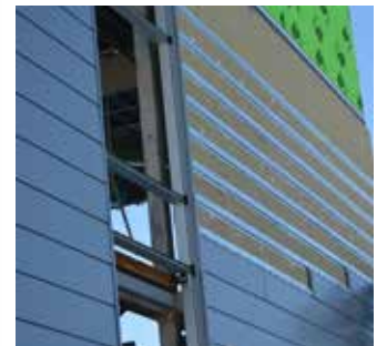
Long screws through horizontal metal hat tracks and rigid ROCKWOOL COMFORTBOARD™ insulation on a commercial building project.
