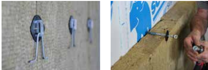
Examples of masonry ties installed through ROCKWOOL CAVITYROCK® insulation.
