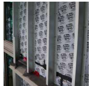
Vertical Z-girt over steel stud wall assembly. Girts are fastened to studs behind at every 16" o.c. resulting in significant thermal bridging through the exterior insulation.
