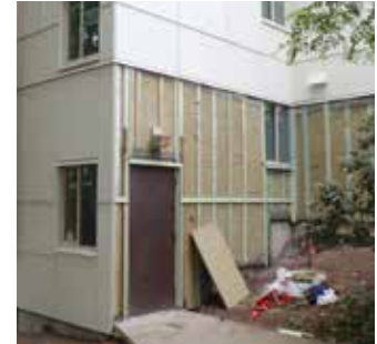
Long screws through vertical wood strapping and rigid ROCKWOOL COMFORTBOARD™ insulation on a multi-family residential project.
