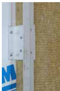
Generic adjustable back to back L-angle clips.
