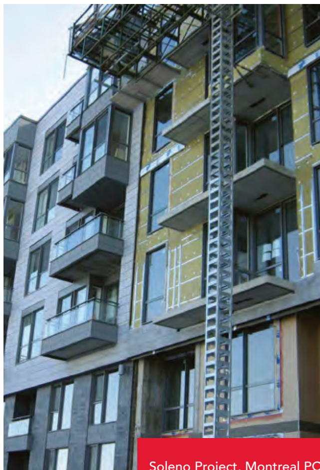
Soleno Project, Montreal PQ ROCKWOOL CAVITYROCK®
