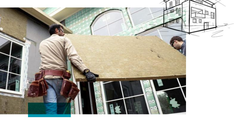
ROCKWOOL Comfortboard<sup>®</sup> 80 thermal insulated sheathing is a rigid stone wool insulation board designed for use as an exterior continuous insulation. Comfortboard<sup>®</sup> 80 does not produce smoke or propagate flames, keeping occupants safe and reducing property damage in the event of a fire. Vapor permeable, this solution allows fast outward drying, keeping moisture out of your wall assembly.
