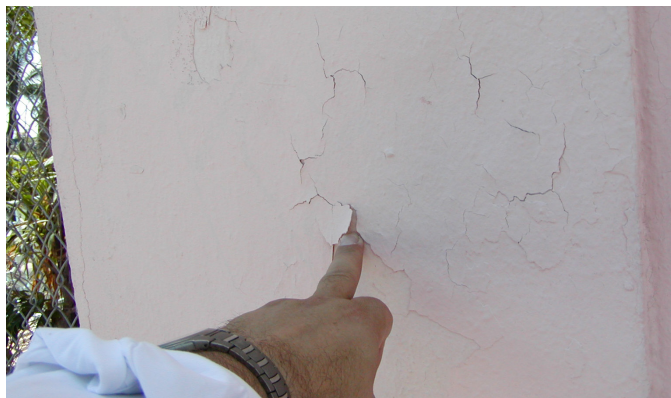
Photograph 1: Impermeable Paint - If the paint on the stucco is too impermeable it bubbles, blisters and peels. The paint on the stucco needs to be greater than 10 perms "wet cup" or it will bubble, blister and peel.
