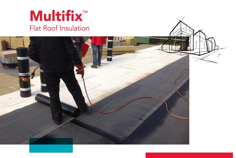
ROCKWOOL Multifix™ is the first stone wool insulation product with a mineral-coated fiberglass facer that is compatible with multiple attachment methods including torched, hot-mopped, cold-adhered and liquid systems.
