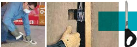
It cuts quickly and accurately with a serrated knife, such as a bread knife, so you can easily achieve optimal fit around pipes, electrical boxes, wiring, ductwork, and between studs and joists that are less than a standard width.
